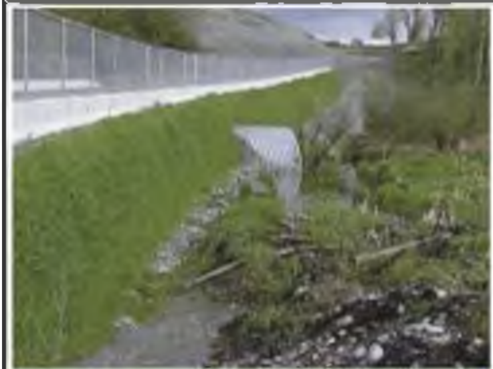
Vegetated Culvert Headwalls
